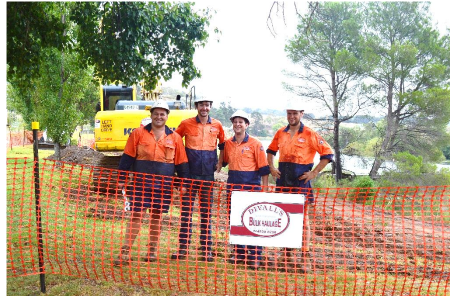
PICTURED ABOVE: STAN WILLIAMS (BOBCAT OPERATOR), MATTHEW BELL (LABOURER), PEDRO VENDEMIATTI (PROJECT ENGINEER) & STEPHEN ARNALL (EXCAVATOR OPERATOR)
