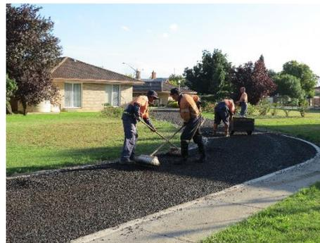
There are also many benefits of a Bituminous Spray Seal which include less greenhouse gases produced in the application of a spray seal as opposed to hot mix, most cost effective treatment for resurfacing roads, a bituminous spray seal is more flexible and can resist fatigue cracking as well as providing a waterproof wearing surface.
